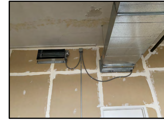
WALL AT MONUMENTAL STAIR LOOKING SOUTH (EXIST. PHOTO)
