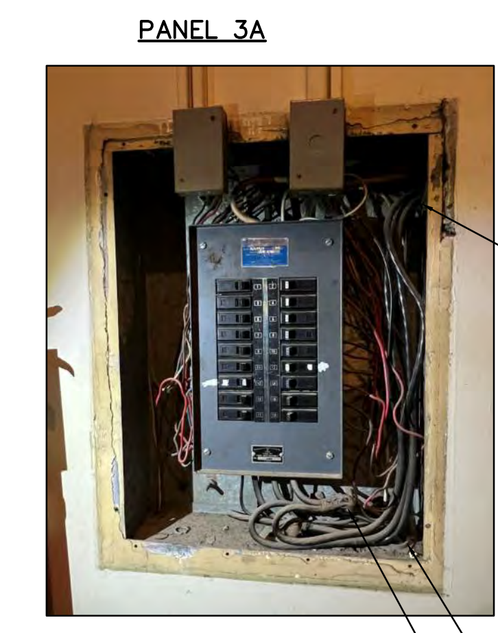
PANEL 3A FEEDER TO PANEL 4A FEEDER FROM MSB FEEDER SPICE ALT.-H2 NOTES
