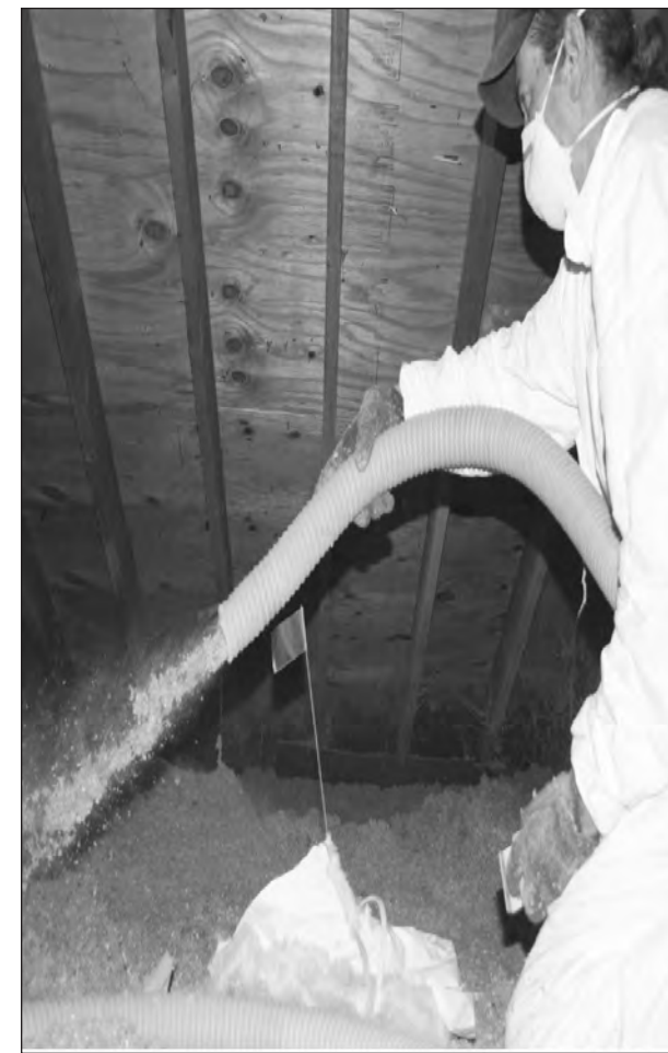
A HAPCAP employee blows insulation into an attic in Murray City. In 2011, 267 homes were weatherized in Murray City as part of a city-wide pilot program.
